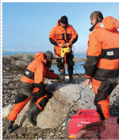
Josef Stemberk, Filip Hartvich and Jan Blahůt installing GNSS measuring place in Hornsund fjord, Svalbard. GNSS measurement campaigns are used to monitor regional tectonic movements and isostatic uplift of the Hornsund fjord area. Photo M. Hladká.
