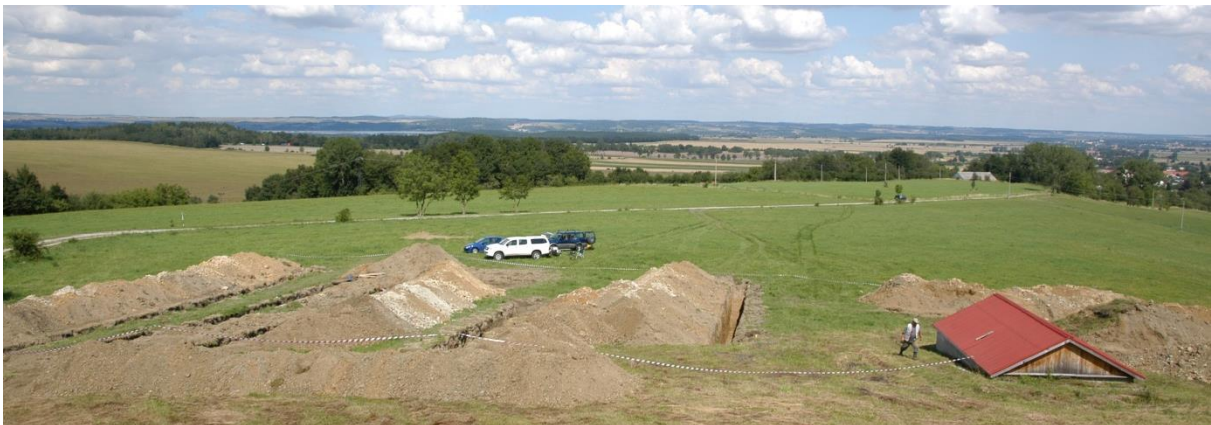
Fig. 1. Bílá Voda trenching site at Sudetic Marginal Fault where late Pleistocene faulting was proved.
